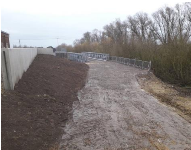
Bridge installation at Welches Dam
