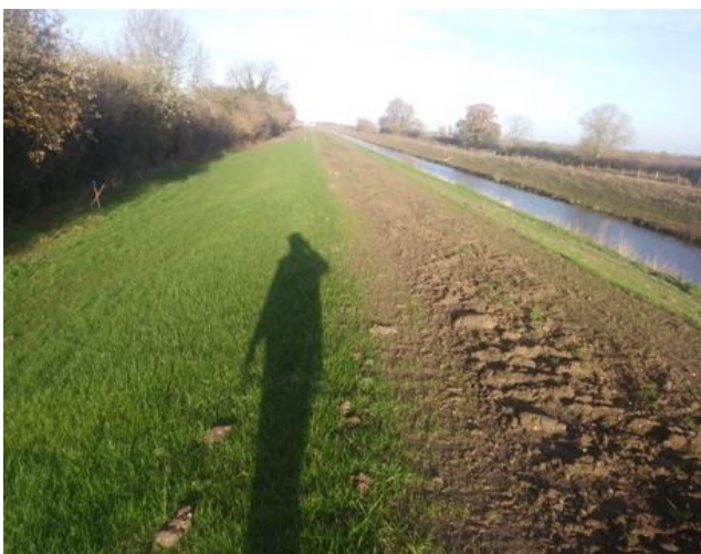
Finished bank profile
