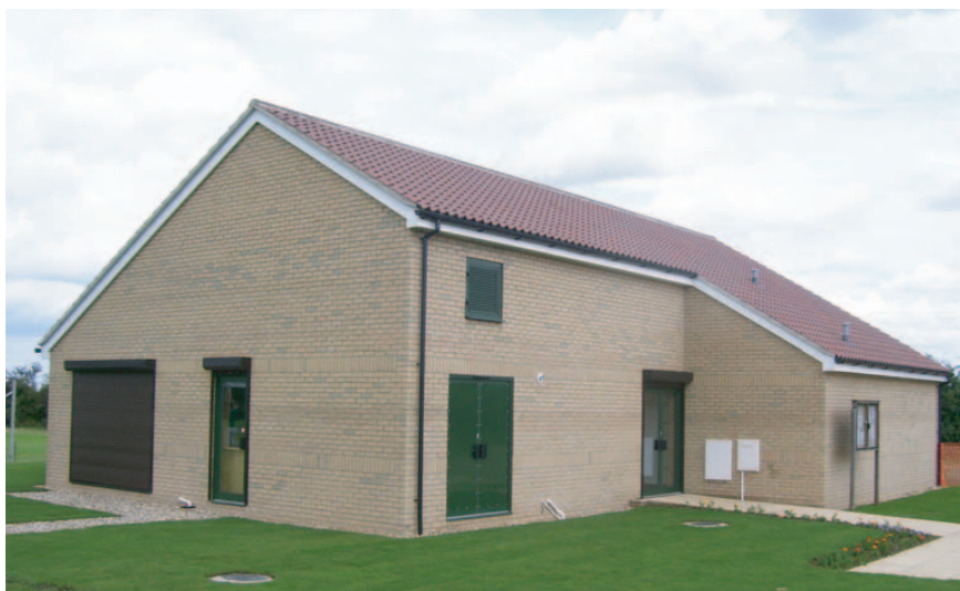
Community Pavilion opened July 2007. A £275k project completed within budget. Supported and funded by Mepal Sports Action Group, The Football Foundation, East Cambridgeshire District Council, WREN, the Grant Weston Trust, Cambridgeshire ACRE and Donarbon.
